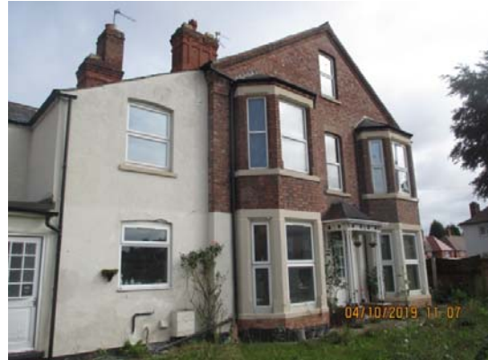
South west (side) elevation of main house
