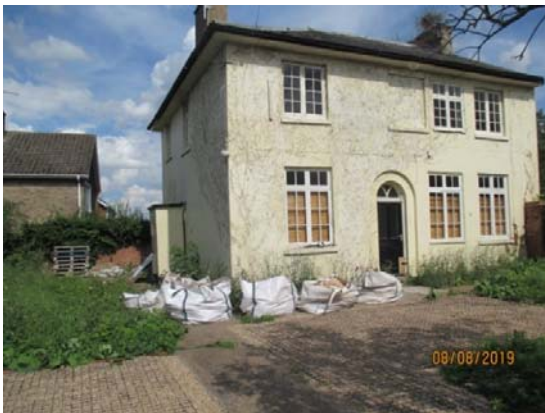
Front elevation of 45 Town Street
