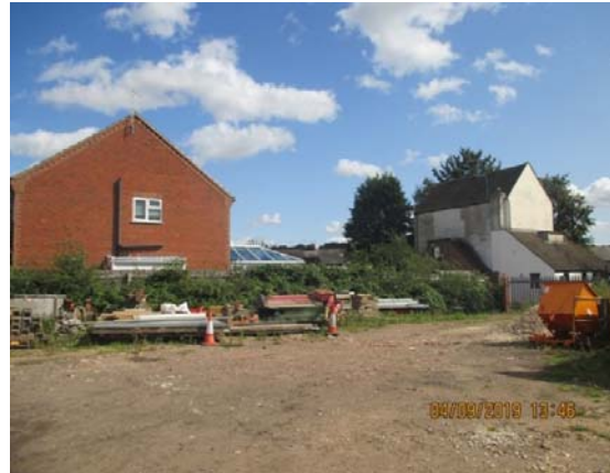
West elevation of no. 6 Meadow View
